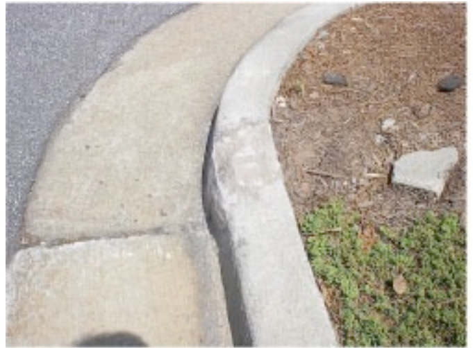
Repair Patched with SR2K
