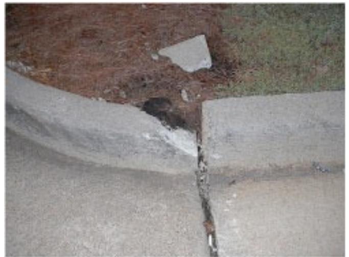
Repair Patched with SR2K
